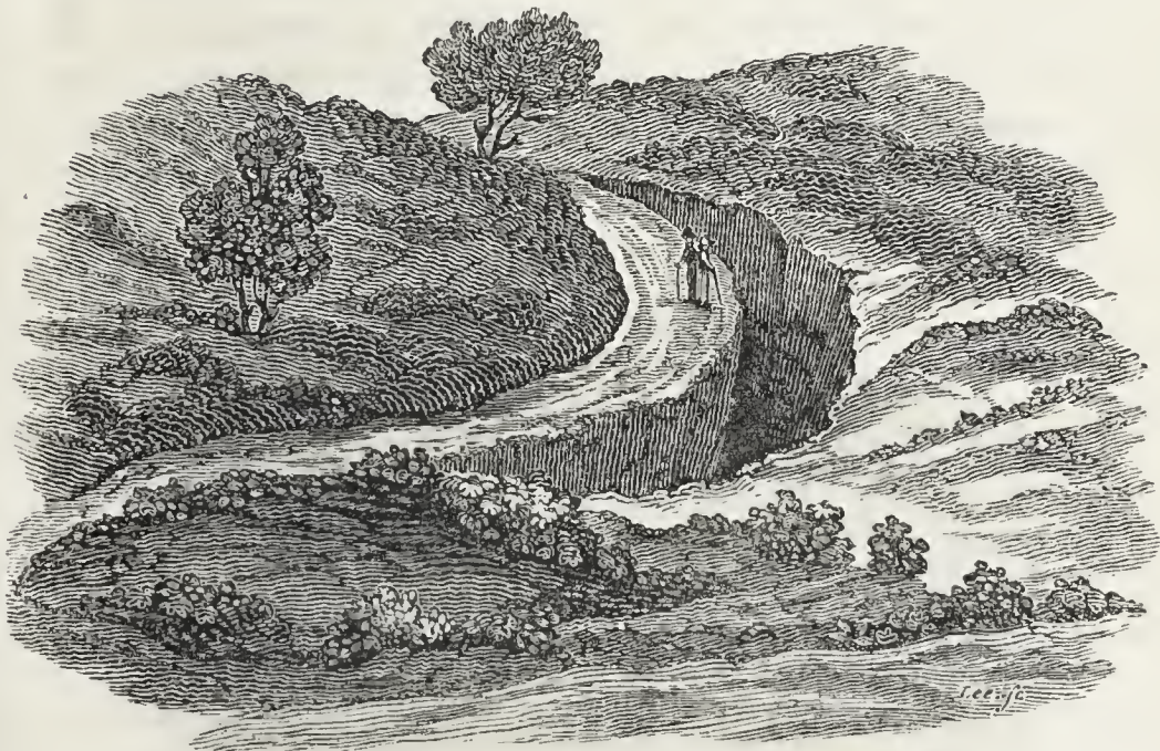
Chasm in the hill of St. Angelo, near Soriano, in Calabria, caused by the earthquake of 1783.
